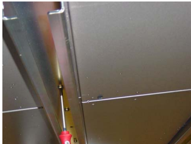
Figure 28. Attaching a unit to the rails from below
