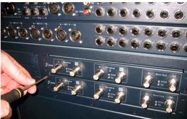
Securing the Snake card to the back panel of the FOH Rack
